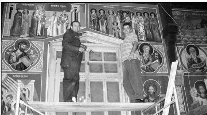
Instalarea ferestrelor/ Window installation - 2005 Părintele/Father Ioan Bunea & Dumitru Borcan
